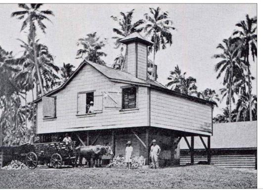
After Kapitan Hufnagel had proved the concept of, what became known in Samoa as, "hot air drying" of copra, it was picked up by most other large coconut plantations, including the two other DH & PG operations at Vaitele and Mulifanua. The latter was the company's biggest plantation at over 5,000 acres and reportedly had several hot air driers, one of which is shown at left.
